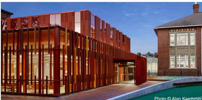
Hyde-Addison Elementary School, Washington, DC
